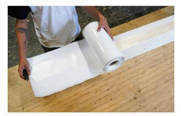
If the overlap occurs at a corner fold, it should preferably rest on membrane already applied rather than directly on the timber, to ensure better sealing and continuity of the protective system.
