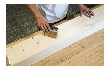
Before gluing, thoroughly clean the surface, which must be smooth, cohesive and free from irregularities. Any surface damage must be assessed and properly treated before laying the membrane.
