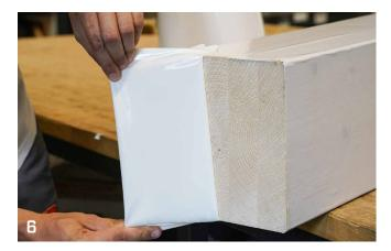
For optimal performance, the membrane should not be directly exposed to weathering and UV rays for more than 8 weeks.
