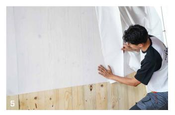
Remove DEFENCE ADHESIVE REMOVABLE. Within 8 weeks if exposed directly to weathering and UV rays.
