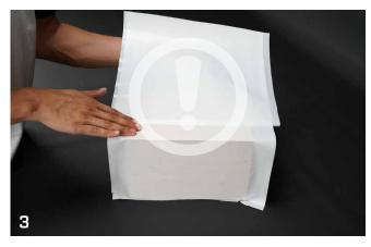
**IMPORTANT**: the product cannot be repositioned on timber. It should not be removed and reapplied, as its adhesive strength would be compromised.
