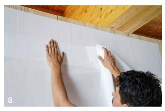
For optimal performance, the membrane should not be directly exposed to weathering and UV rays for more than 8 weeks.
