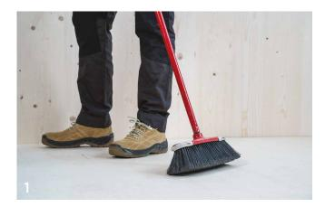
Before gluing, thoroughly clean the substrate, removing any dust, residue and surface impurities that could compromise the membrane's adhesion.
