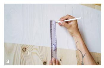
Before applying DEFENCE ADHESIVE REMOVABLE, ensure an overlap of 10–15 cm starting from the base of DEFAREM360.
