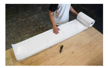
Accurately position the membrane on the surface, ensuring proper alignment and full coverage of the area to be treated before gluing.
