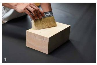
Before gluing, thoroughly clean the surface, which must be smooth, cohesive and free from irregularities. Any surface damage must be assessed and properly treated before laying the membrane.
